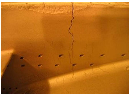
Fig. 7 1.5 mm wide cracks on the sidewalls of a typically industrial gas turbine nozzle segment
